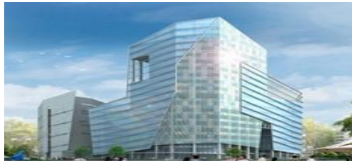
Fusionopolis Phase 2A To Complete in 2015
