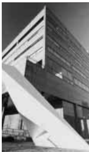
The Federal Reserve Bank of Philadelphia was the site of the conference on the euro.
